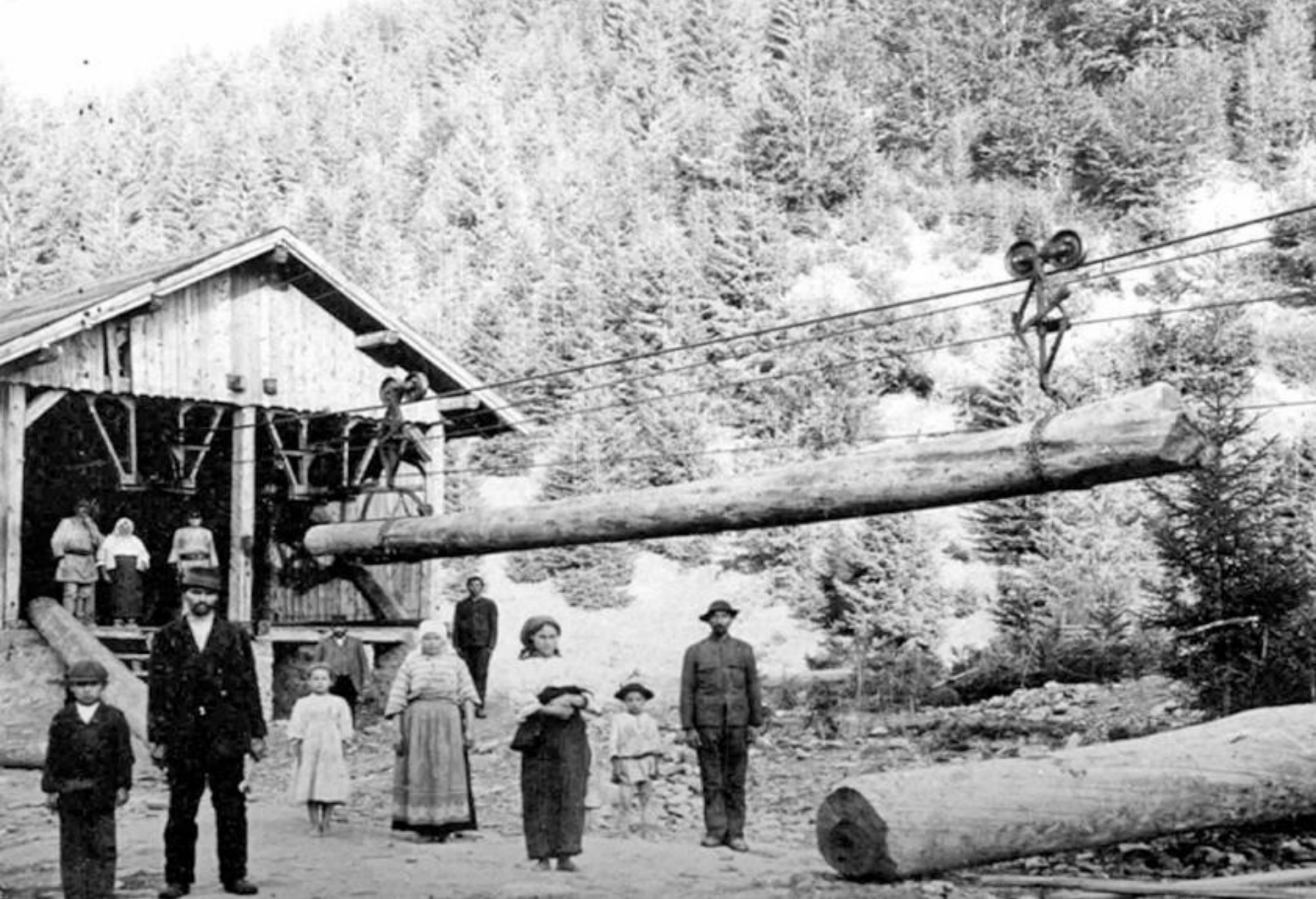
Air transportation of timber with cables in “Gournosovo” area, beginning of the 20 th century.
